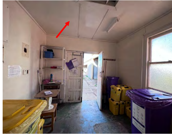
Photo 68: Old Morgue – Internal assumed asbestos fibre cement ceiling lining
