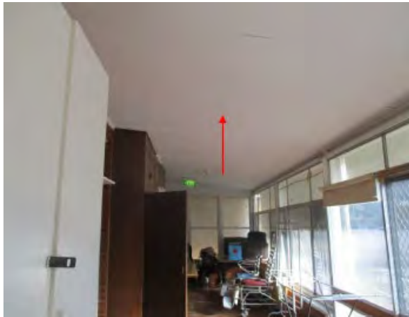
Photo 16: Wentworth Hospital Services - Internal Former Maternity west & north-west veranda asbestos ceiling lining
