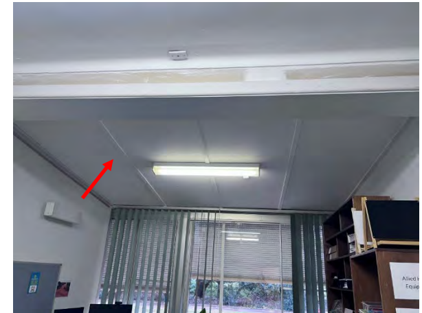
Photo 18: Wentworth Hospital Services - Internal northern 'NUM's office' asbestos ceiling lining
