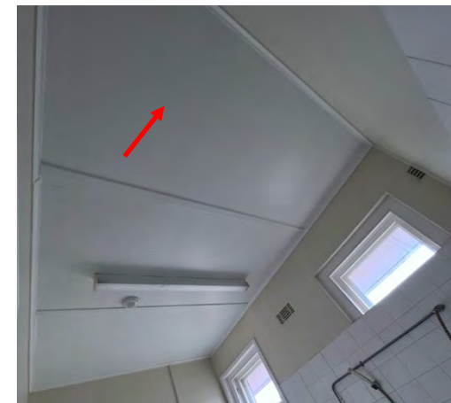
Photo 108: Senior Centre – North-eastern bathroom asbestos ceiling lining
