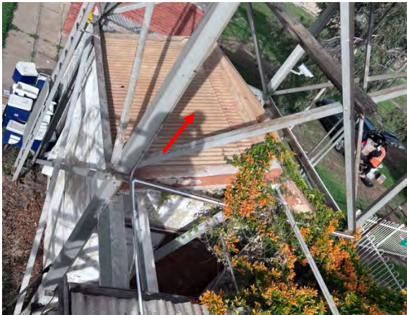
Photo 52: Pump Shed – Asbestos super 6 roofing
