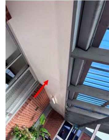
Photo 33: Wentworth Hospital Services - External flat sheet asbestos eaves - Internal Courtyard
