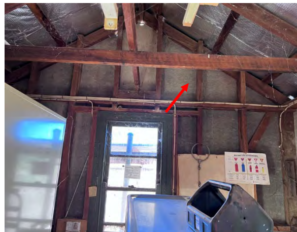
Photo 65: Maintenance Storage Shed – External asbestos cladding and silver sarked roof
