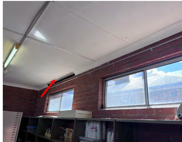
Photo 26: Wentworth Hospital Services - Hotel Services Storeroom asbestos ceiling lining
