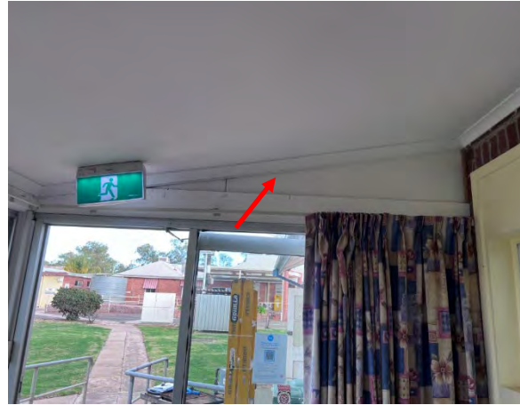
Photo 110: Senior Centre – south-western wall lining above glass door asbestos wall lining
