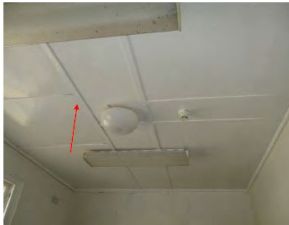
Photo 5: Wentworth Hospital Services – Former Surgical sterile room asbestos ceiling lining
