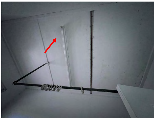
Photo 106: Senior Centre – western bathroom asbestos ceiling lining
