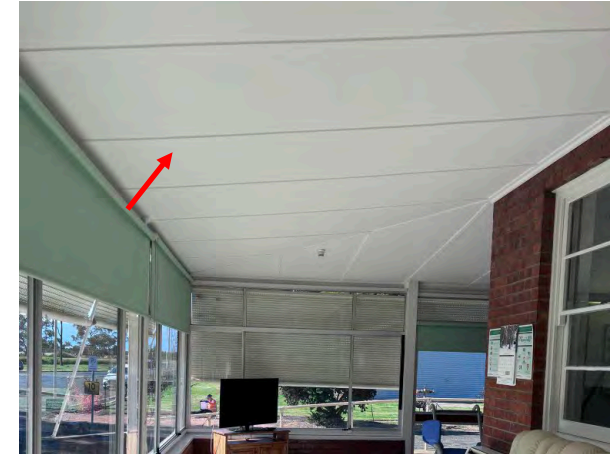
Photo 21: Wentworth Hospital Services - Internal north eastern veranda asbestos ceiling lining
