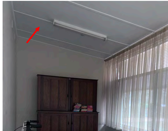
Photo 17: Wentworth Hospital Services – Internal northern 'mental health' asbestos ceiling lining
