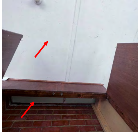
Photo 14: Wentworth Hospital Services - Internal former maternity veranda–asbestos cupboard ceiling lining
