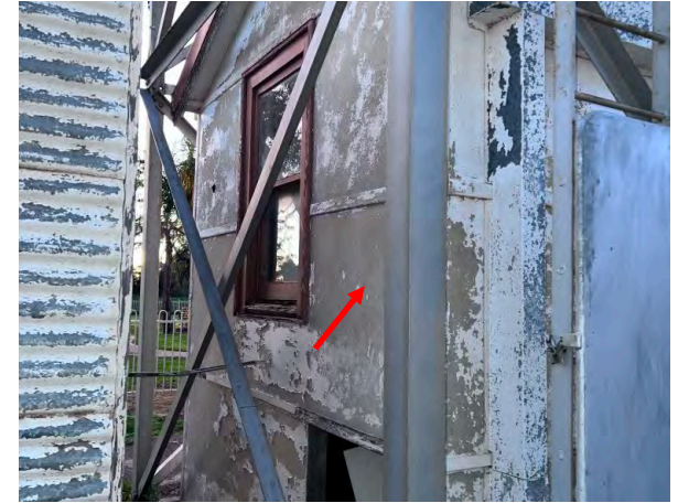
Photo 51: Pump Shed - External asbestos walls fibre cement sheet cladding
