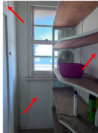
Photo 86: Old Nurses Home – Asbestos fibre cement internal pantry wall lining
