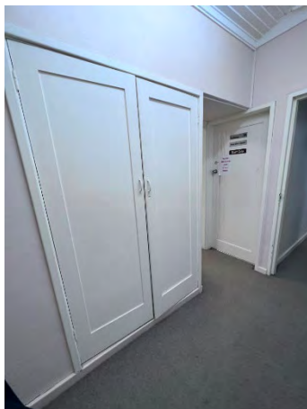
Photo 103: Senior Centre – Internal western corridor storage asbestos cupboard lining
