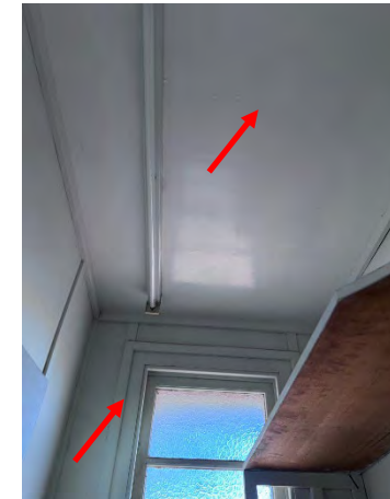
Photo 87: Old Nurses Home – Asbestos fibre cement internal pantry wall & ceiling lining
