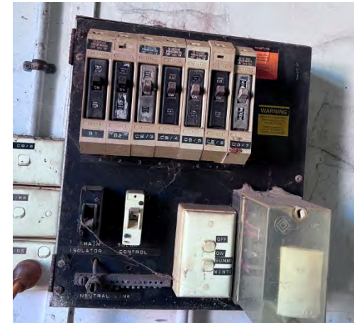
Photo 48: Old Boiler House – Assumed asbestos black backed electrical board
