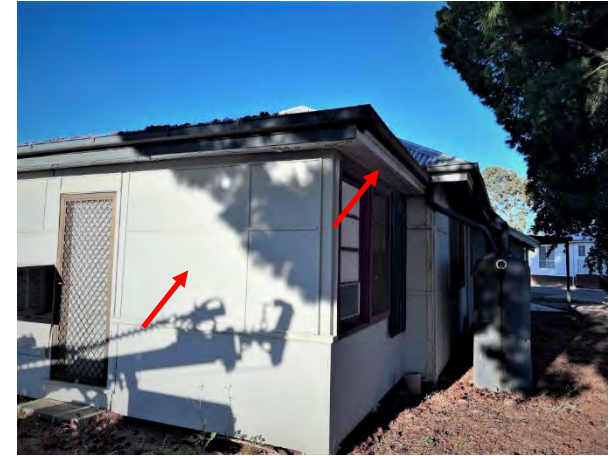
Photo 81: Old Nurses Home – Asbestos fibre cement eaves and external cladding
