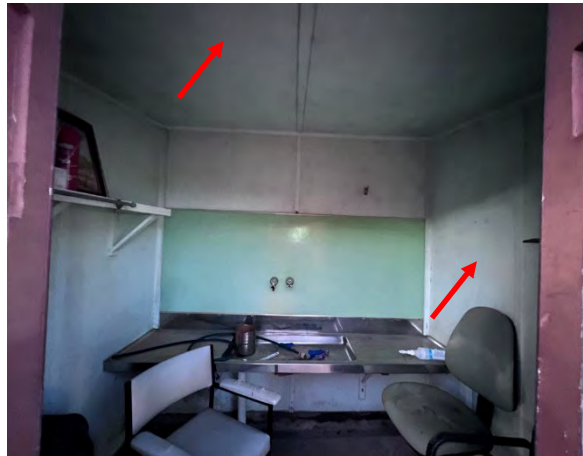
Photo 56: Dirty Linen – Internal asbestos wall and ceiling lining fibre cement sheeting
