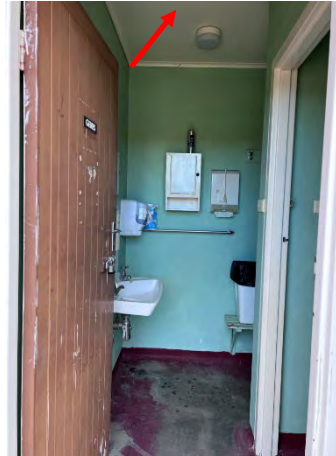
Photo 62: Staff Amenities – Assumed asbestos ceiling linings ceiling and brown lead based paint
