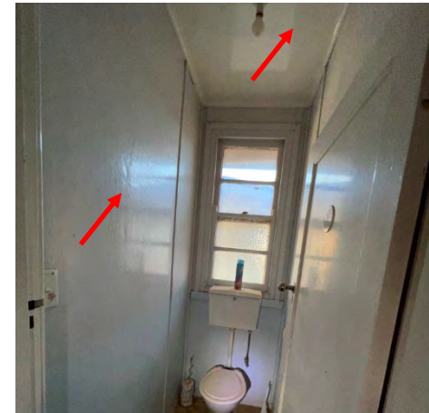
Photo 84: Old Nurses Home – Asbestos fibre cement internal toilet wall & ceiling lining
