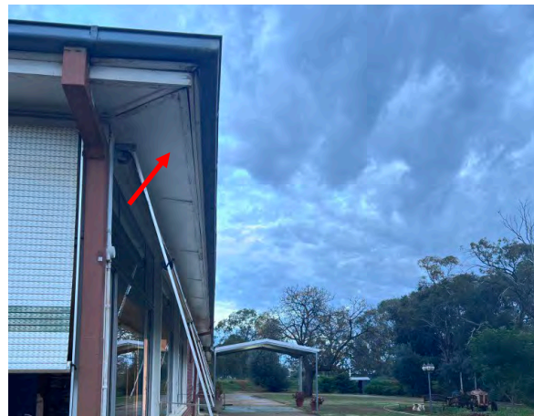
Photo 29: Wentworth Hospital Services - External flat sheet asbestos eaves
