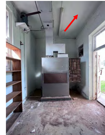
Photo 6: Wentworth Hospital Services – Old Records Room asbestos ceiling lining
