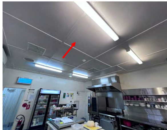
Photo 23: Wentworth Hospital Services - Internal Hotel Services kitchen – asbestos ceiling lining
