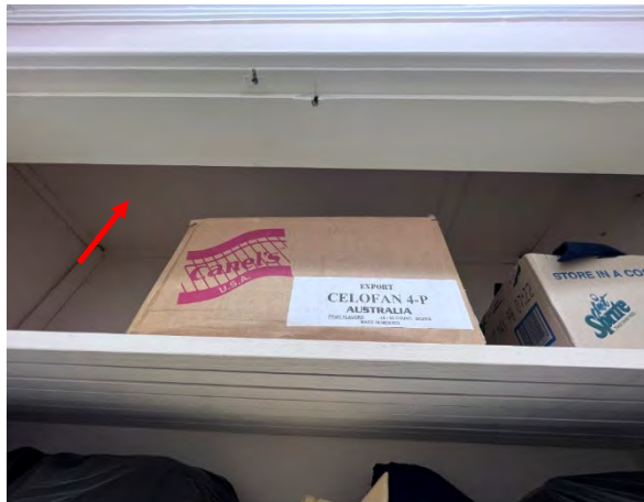
Photo 104: Senior Centre – Internal western corridor storage asbestos cupboard lining
