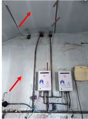
Photo 44: Old Boiler House - Internal asbestos wall and ceiling lining
