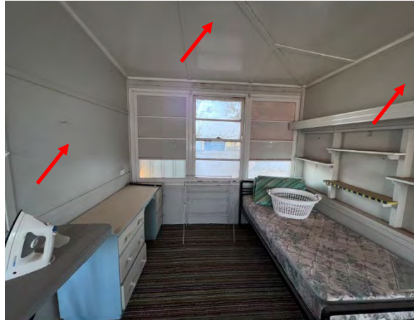
Photo 92: Old Nurses Home – Internal western room asbestos wall and ceiling lining
