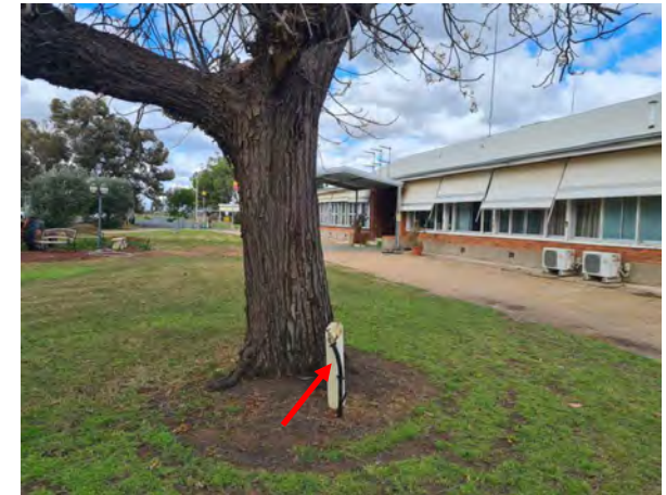
Photo 36: Wentworth Hospital Services - External assumed asbestos containing tap pipe stand
