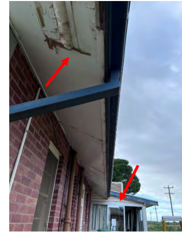
Photo 111: Senior Centre – Asbestos fibre cement eave lining
