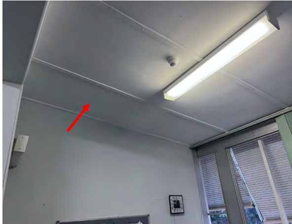
Photo 19: Wentworth Hospital Services - Internal northern 'Nurse Manager' asbestos ceiling lining
