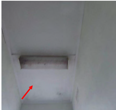
Photo 7: Wentworth Hospital Services - North-western staff bathroom asbestos ceiling lining
