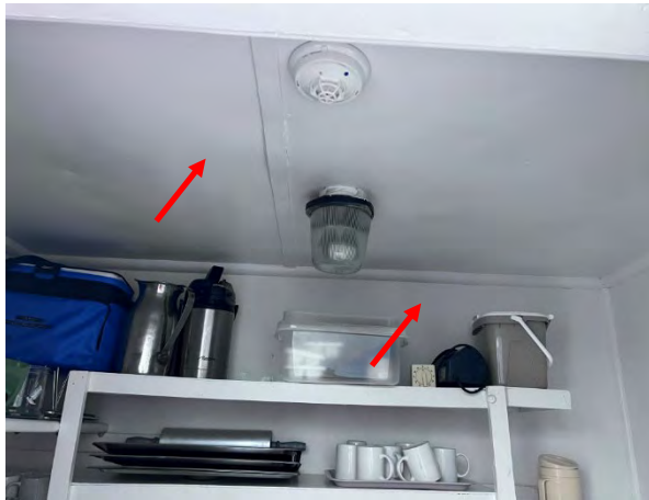
Photo 25: Wentworth Hospital Services - Internal Hotel Services eastern pantry – asbestos ceiling and wall lining
