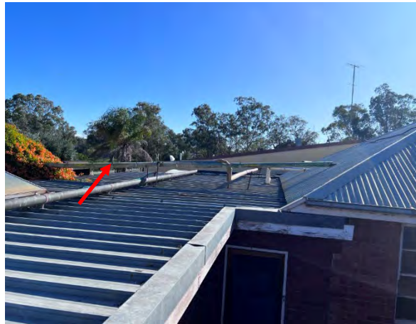
Photo 35: Wentworth Hospital Services - External south-eastern roof assumed asbestos containing lagged pipe
