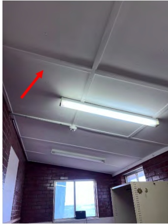
Photo 109: Senior Centre – Eastern storage room asbestos ceiling lining
