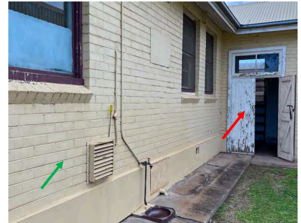
Photo 42: Wentworth Hospital Services - External, Old Records Room timber door white lead paint, Yellow non-lead paint
