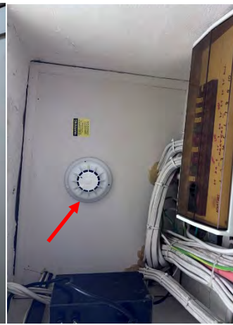
Photo 101: Senior Centre – Internal western corridor communications asbestos cupboard lining
