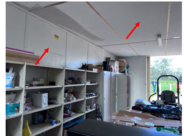
Photo 72: Maintenance Workshop – Internal asbestos fibre cement sheet ceiling and wall lining
