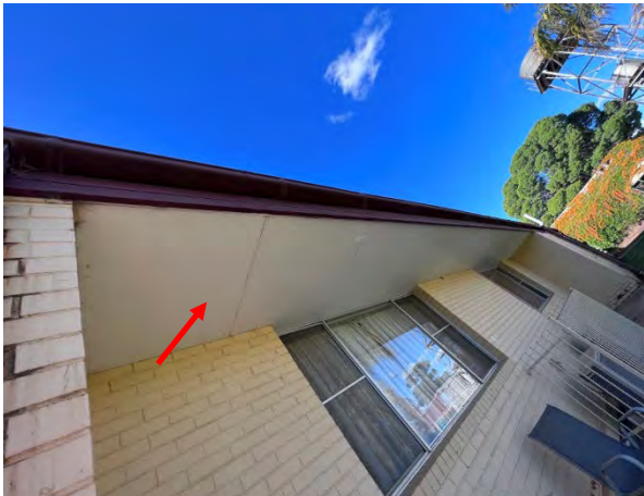
Photo 34: Wentworth Hospital Services - External flat sheet asbestos eaves - southern awning linings
