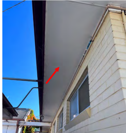
Photo 32: Wentworth Hospital Services - External flat sheet asbestos eaves
