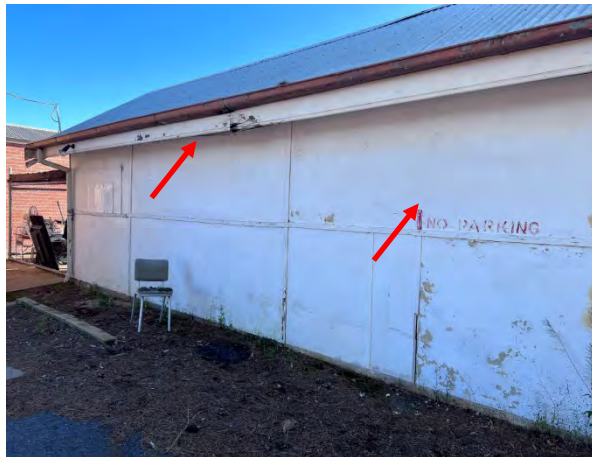
Photo 64: Maintenance Storage Shed - Asbestos fibre cement sheeting eaves & external wall cladding
