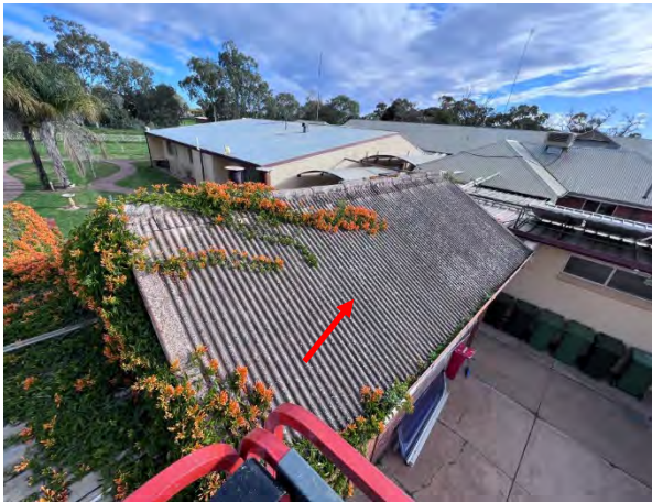
Photo 46: Old Boiler House – Asbestos super 6 Roofing
