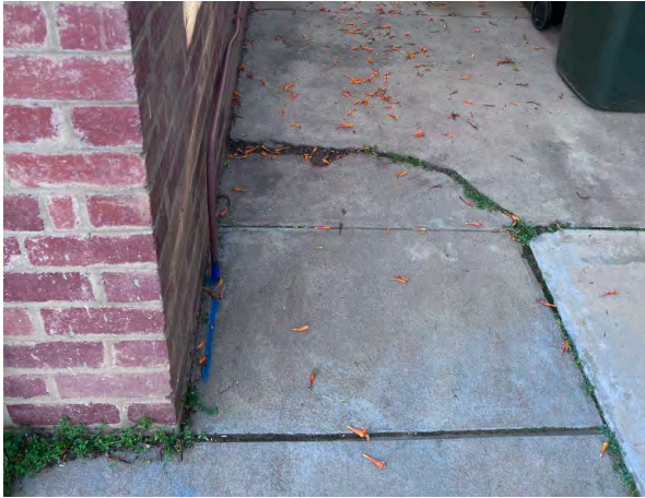
Photo 49: Non-asbestos mastic between buildings 1 & 2
