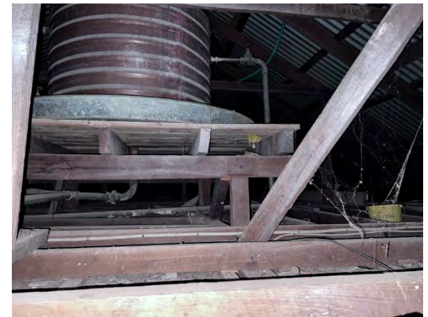
Photo 96: Old Nurses Home – Ceiling Cavity – Assumed asbestos containing former hot water system
