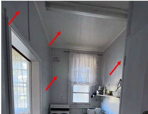
Photo 85: Old Nurses Home – Asbestos fibre cement internal kitchen wall & ceiling lining
