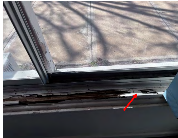
Photo 41: Wentworth Hospital Services - Internal – timber skirting boards, architraves, door jambs and windows White lead paint
