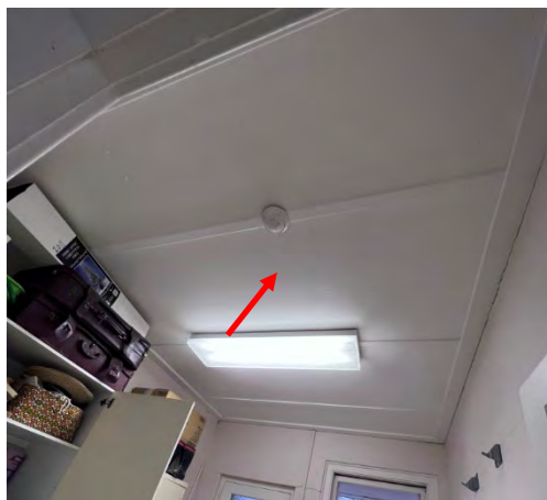
Photo 107: Senior Centre – Laundry asbestos ceiling lining
