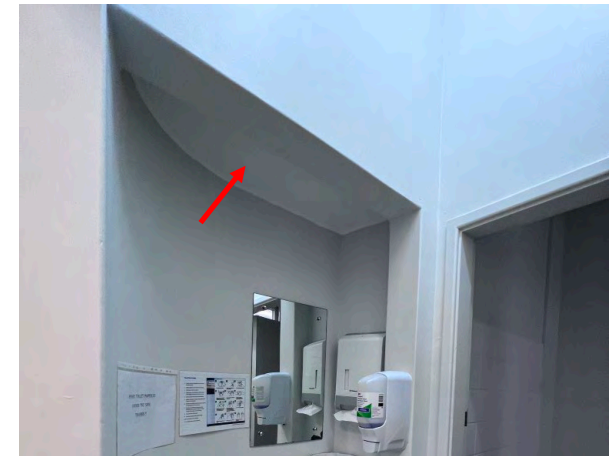
Photo 9: Wentworth Hospital Services - North-western corridor hand wash alcove asbestos ceiling lining
