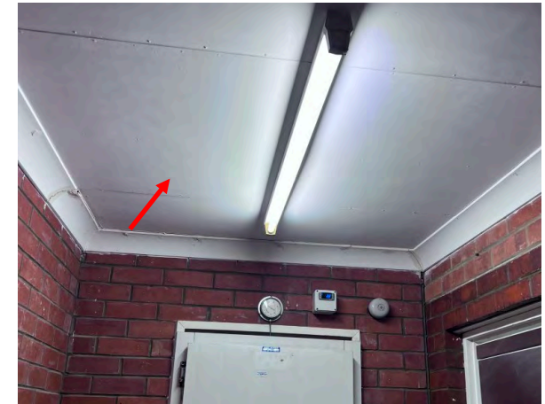
Photo 27: Wentworth Hospital Services - Hotel Services Hallway adjacent Janitors Room asbestos ceiling lining
