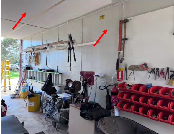
Photo 73: Maintenance Workshop – Internal asbestos fibre cement sheet ceiling and wall lining
