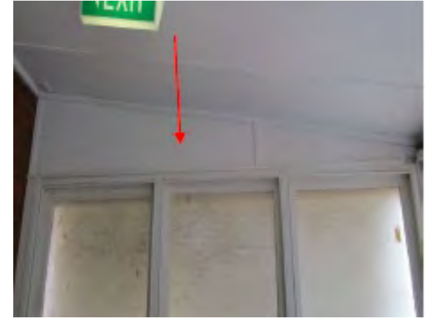
Photo 15: Wentworth Hospital Services - Internal former maternity veranda lining – south-west asbestos wall lining
