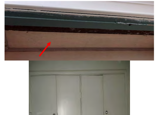
Photo 12: Wentworth Hospital Services - Internal, Former Maternity hallway asbestos cupboard ceiling lining
