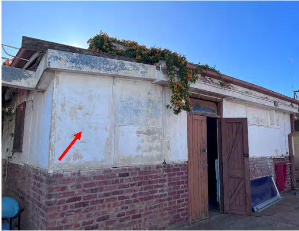
Photo 43: Old Boiler House – Old Boiler House Overview & External asbestos cladding with brick lower
