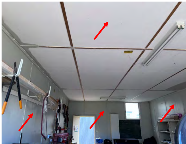
Photo 70: Maintenance Workshop – Internal asbestos fibre cement sheet ceiling and wall lining
