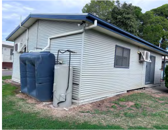
Photo 98: University Staff Quarters – East external hot water system
