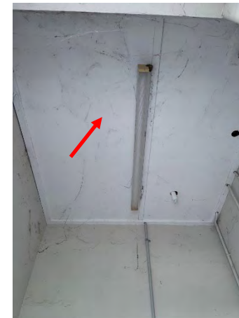
Photo 105: Senior Centre – South-western storeroom asbestos ceiling lining
