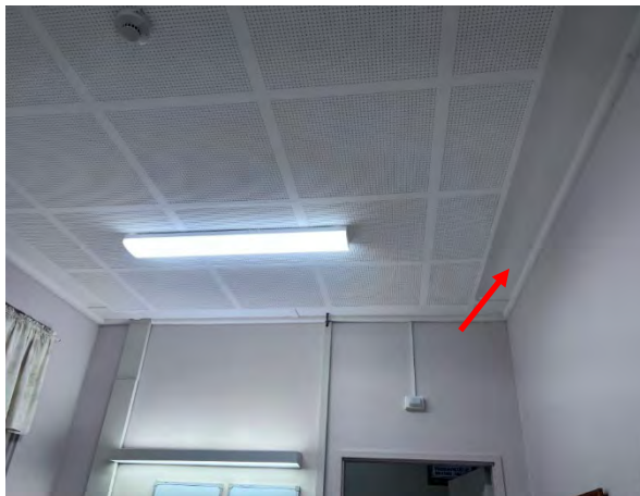
Photo 10: Wentworth Hospital Services - Northern Palliative Care asbestos ceiling lining
