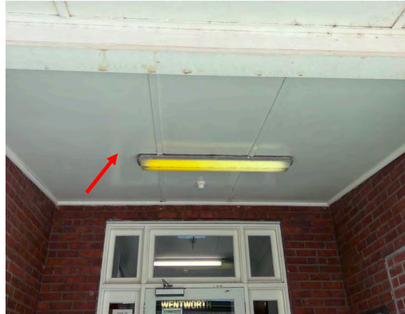
Photo 20: Wentworth Hospital Services - External northern entrance porch asbestos ceiling lining
