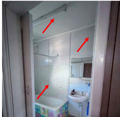
Photo 83: Old Nurses Home – Asbestos fibre cement internal bathroom wall & ceiling lining
