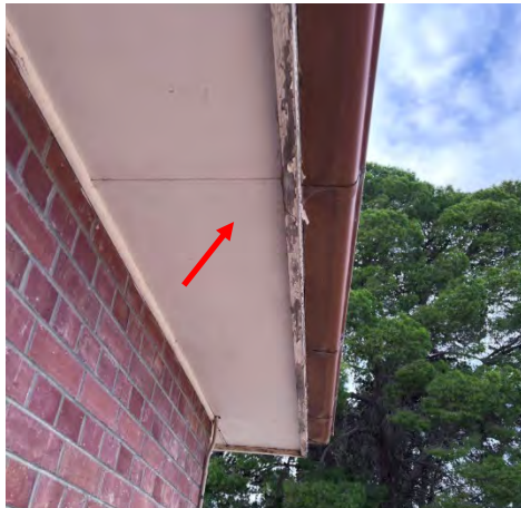
Photo 61: Staff Amenities – Asbestos fibre Cement Sheet eaves
