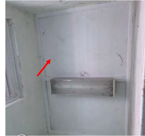
Photo 3: Wentworth Hospital Services - Former Maternity Bathroom Asbestos Ceiling Lining
