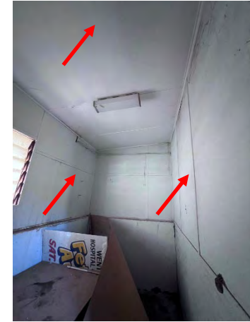
Photo 45: Old Boiler House - Internal asbestos wall, ceiling lining & joining battens
