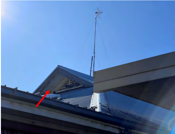
Photo 31: Wentworth Hospital Services - External flat sheet asbestos eaves & gables
