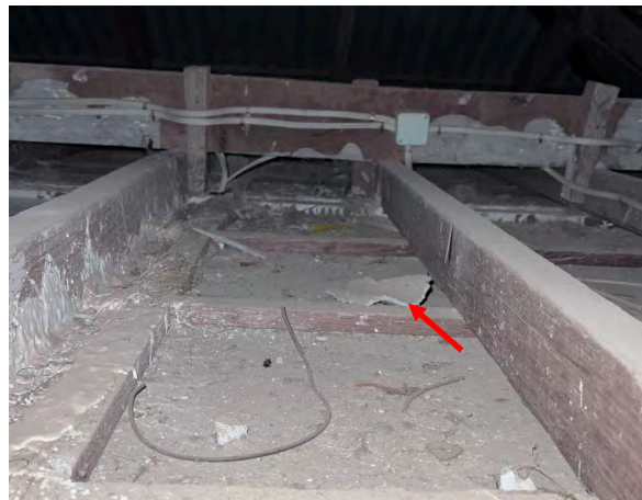
Photo 89: Old Nurses Home – Ceiling cavity, Accessed through kitchen – broken asbestos super six sheeting
