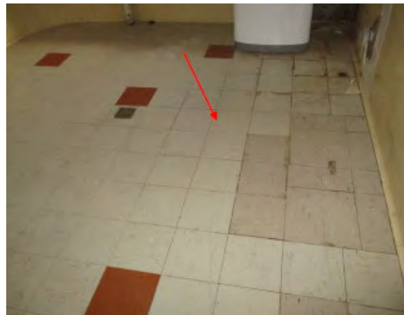
Photo 11: Wentworth Hospital Services - Former Maternity Pan Room asbestos flooring
