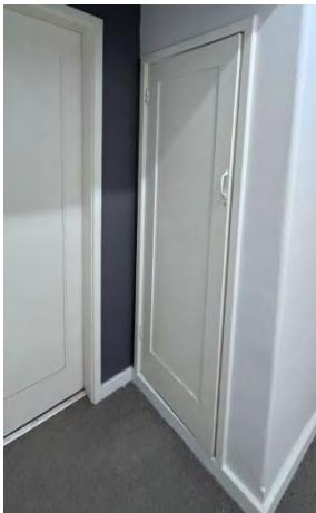
Photo 100: Senior Centre – Internal western corridor asbestos cupboard lining
