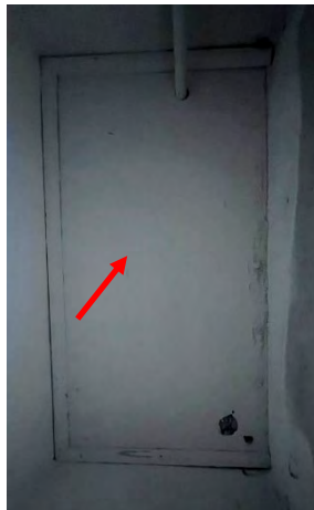
Photo 100: Senior Centre – Internal western corridor asbestos cupboard lining
