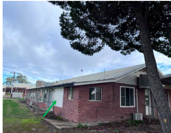
Photo 113: Senior Centre – Non-asbestos south-eastern cladding facade
