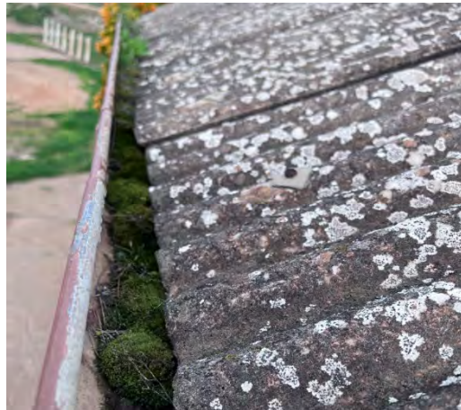
Photo 47: Old Boiler House – Asbestos super 6 Roofing and Gutter Debris
