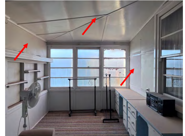
Photo 93: Old Nurses Home – Internal western room asbestos wall and ceiling lining
