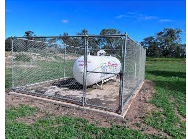
Photo 117: Building 16 – LPG gas storage
