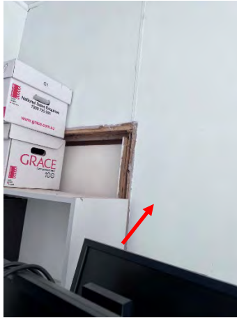
Photo 13: : Wentworth Hospital Services – Internal former maternity west veranda asbestos wall lining
