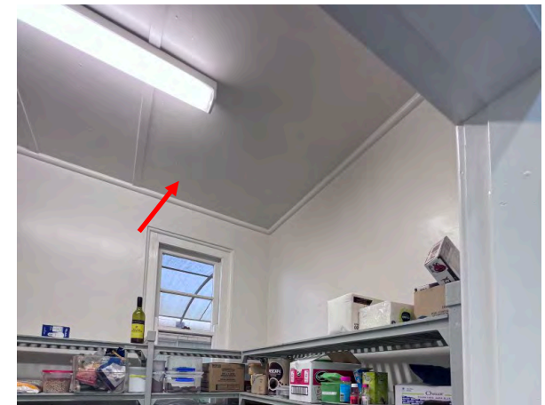
Photo 24: Wentworth Hospital Services - Internal Hotel Services western pantry – asbestos ceiling lining
