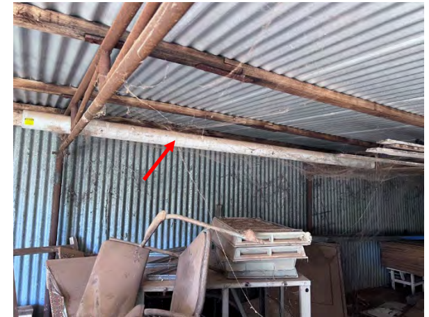
Photo 78: Carports/Storage Sheds – Assumed asbestos fibre cement pipe in rafters of shed
