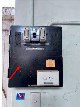
Photo 38: Wentworth Hospital Services - Old Records Room – southern wall – assumed asbestos electrical backing board
