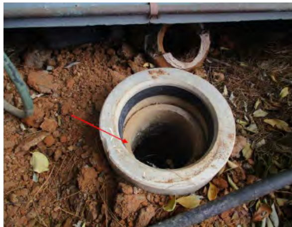
Photo 95: Old Nurses Home – External east – assumed asbestos containing gully drain pipe
