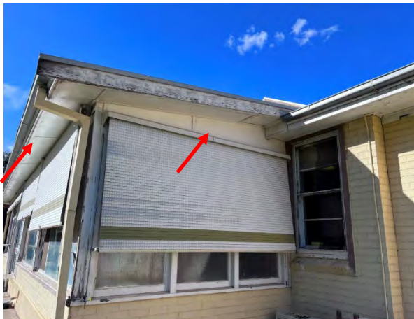
Photo 28: Wentworth Hospital Services - External asbestos flat sheet eaves
