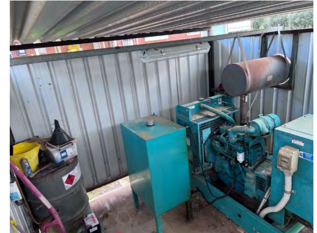
Photo 75: Emergency Generator Shed – Generator Machinery, assumed asbestos gaskets
