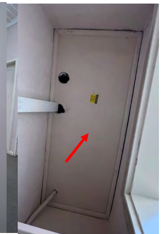
Photo 102: Senior Centre – Internal western corridor communications asbestos cupboard lining
