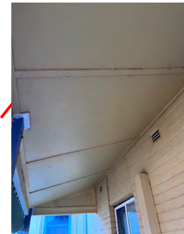
Photo 30: Wentworth Hospital Services - External flat sheet asbestos eaves – Internal courtyard
