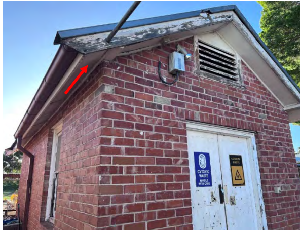
Photo 67: Old Morgue – Asbestos fibre cement eaves
