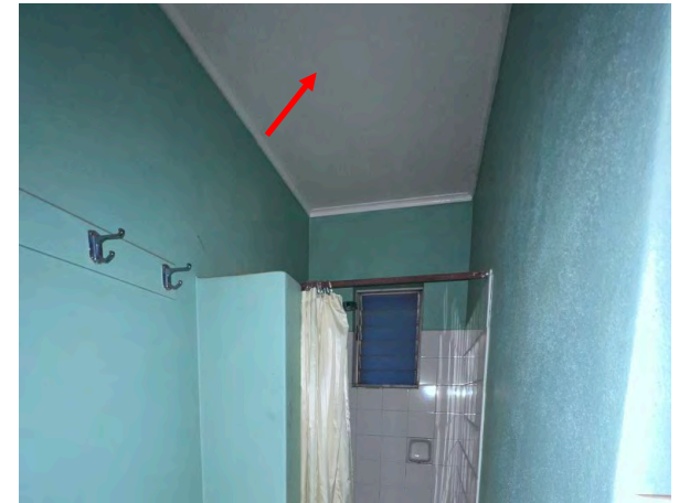
Photo 63: Staff Amenities – Assumed asbestos ceiling linings
