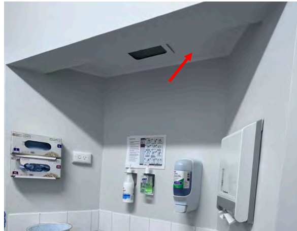
Photo 8: Wentworth Hospital Services - North-western staff bathroom alcove asbestos ceiling lining
