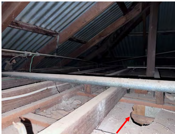
Photo 88: Old Nurses Home – Ceiling cavity, Accessed through kitchen – broken asbestos fibre cement sheeting
