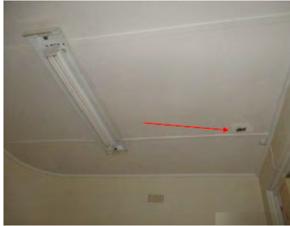
Photo 2: Wentworth Hospital Services – Asbestos containing FCS to ceiling of Former Maternity Pan RoomFormer Maternity Bathroom Ceiling Lining
