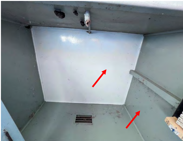
Photo 82: Old Nurses Home – Asbestos fibre cement external cladding & assumed porch lining
