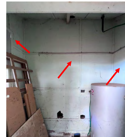
Photo 90: Old Nurses Home – Internal of southern plant room – asbestos fibre cement sheet wall lining
