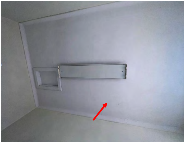
Photo 4: Wentworth Hospital Services - Former Surgical change room asbestos ceiling lining
